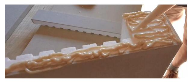
1. APPLIQUER NOTRE COLLE D4 SUR LES SURFACES DE CONTACT DES MODENATURES OU APPUIS ENDOMMAGES.
